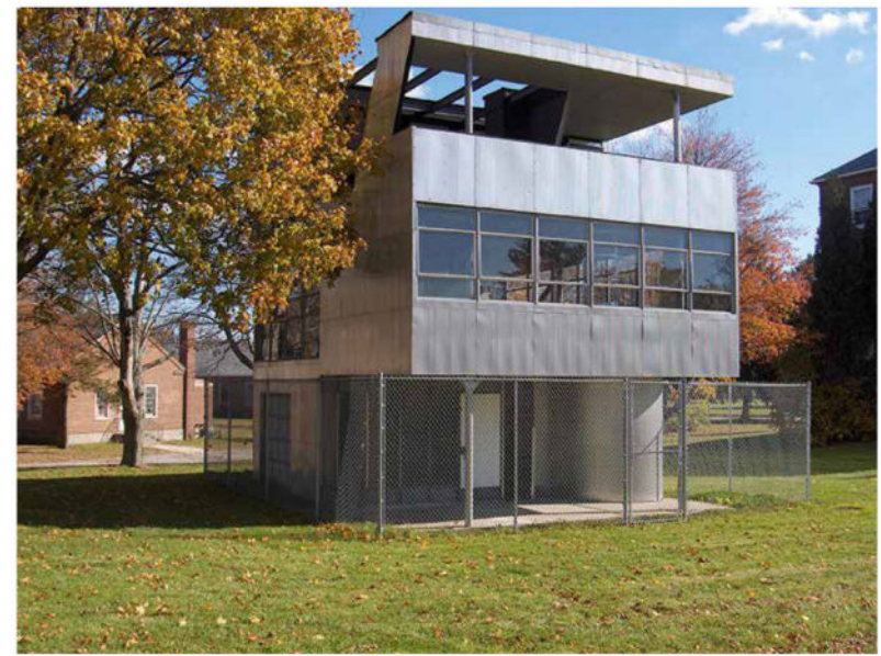
4-42 Enclosed - 2000 4-43 Enclosed 4-44 Enclosed 4-45 Enclosed
